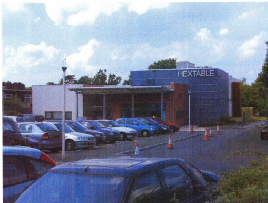
VIEW FROM SOUTH-EAST LOOKING TOWARDS MAIN ENTRANCE
